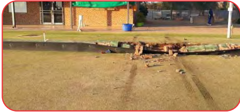
DAMAGE: The green at Groblersdal BC, showing damage after idiots ran a bakkie through it
